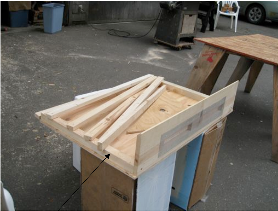
Bottom with 2x2 at base (could be made from two 1x2s).
